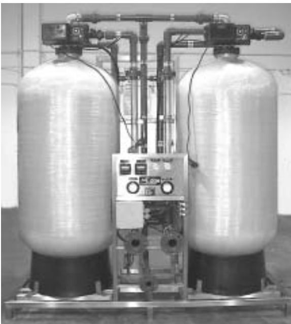
FIGURE 12: Typical Sorption System Composed of Pressure Vessels with Iron-based Sorption Media Capable of Treating 100 gpm (AdEdge Technologies, Inc., Norcross, Georgia)
